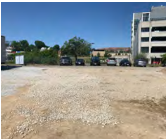
Install a construction access pad
