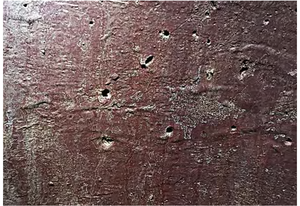
West Tank Side Wall. Pitting Observed
