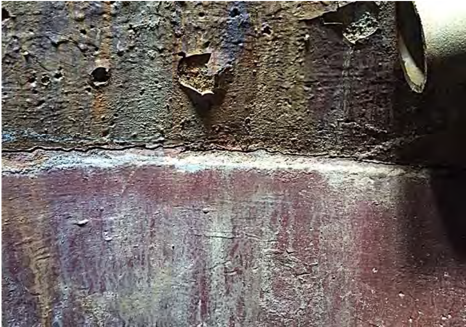
West Tank Sidewall. Crack Observed at Seam
