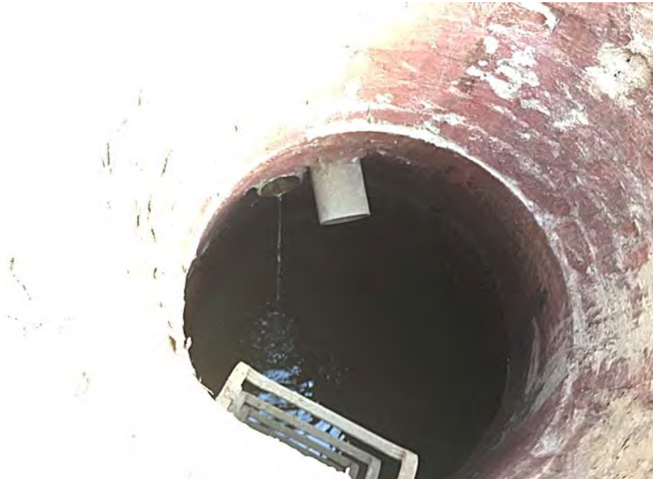
Flow Observed From Drain to Tank
