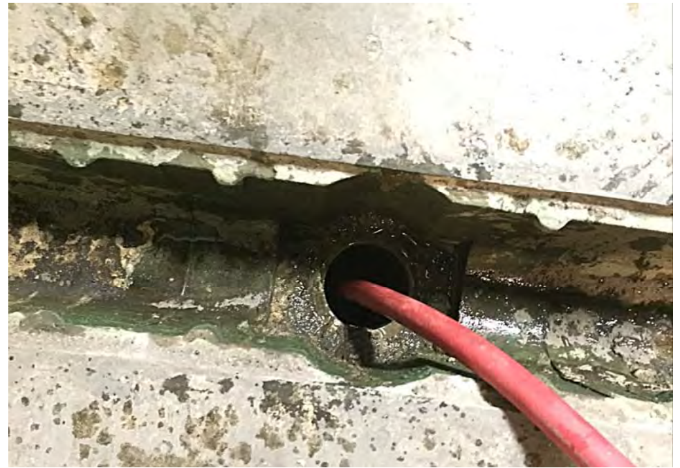
Drain Jetting Process
