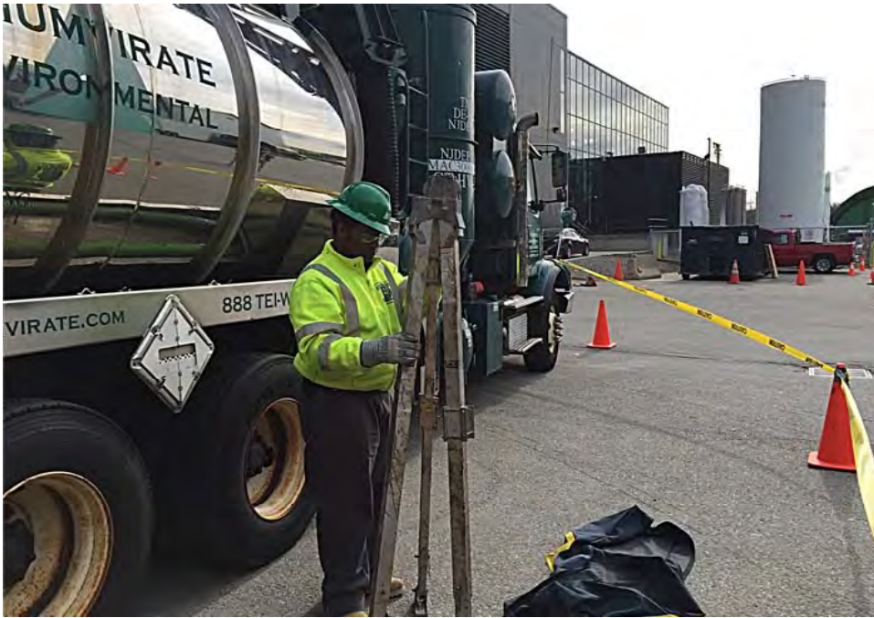
Confined Space Entry Set-Up
