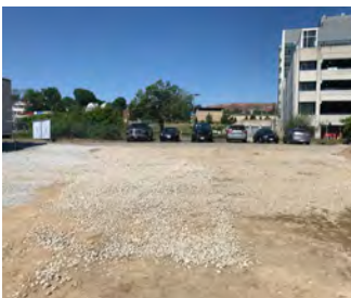
Install a construction access pad
