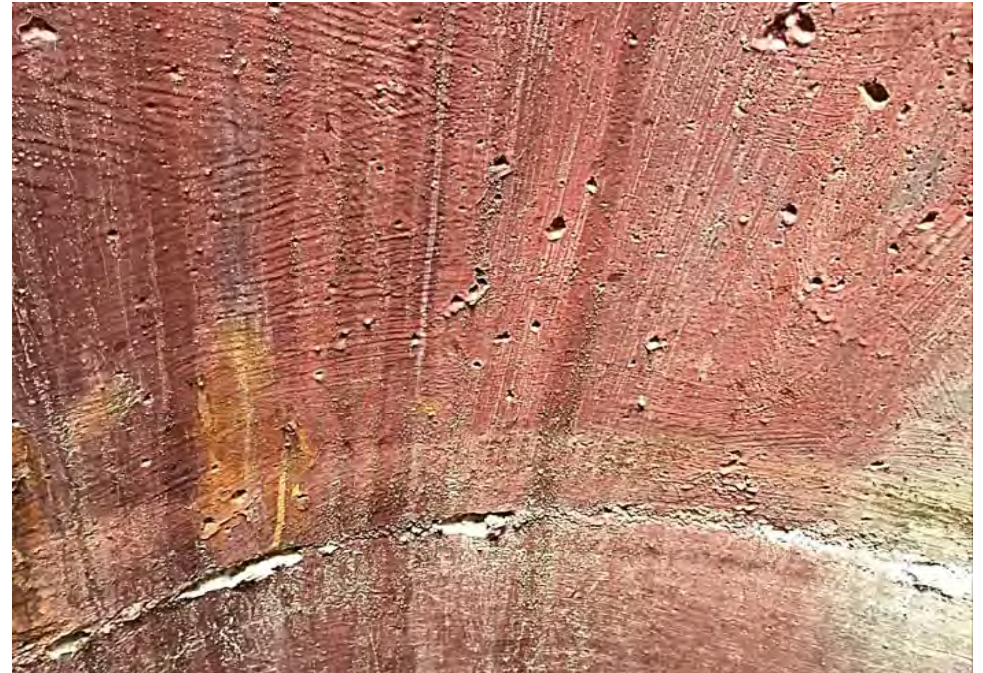
East Tank Walls With Minor Cracks and Pitting
