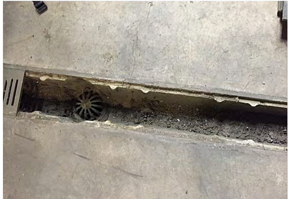
Trench Drain Before Cleaning
