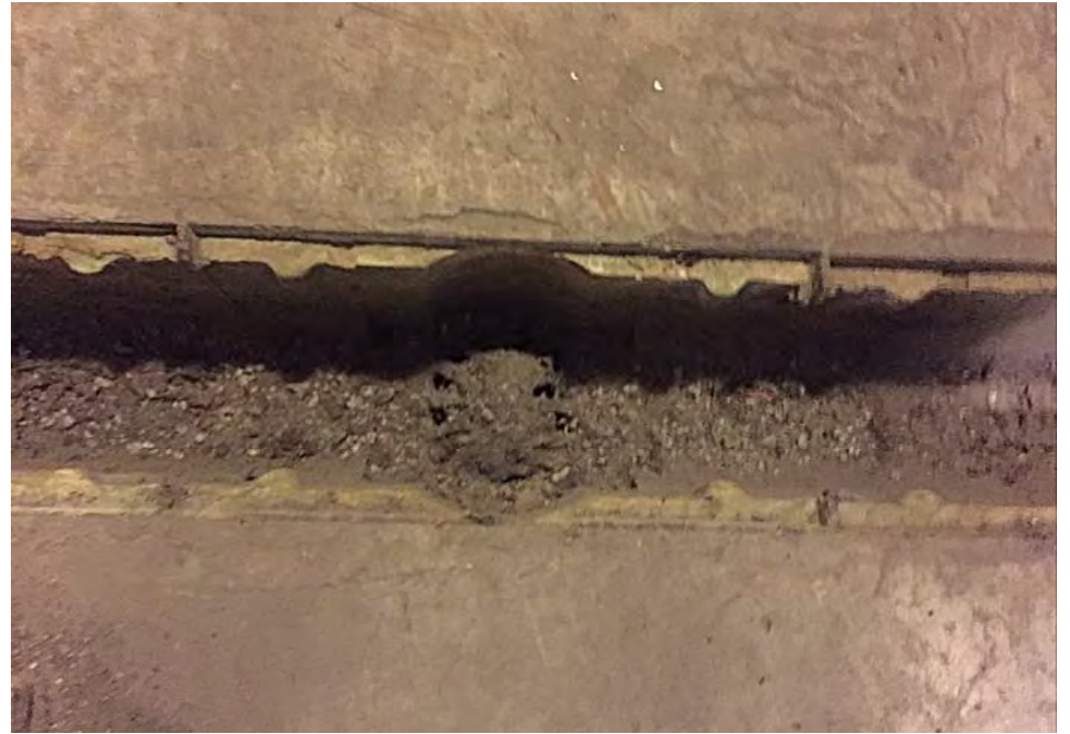
Trench Drain Before Cleaning
