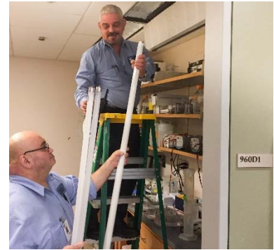
Installation of LEDs in the Lazare Research Building
