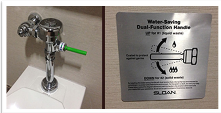
Figure 1 Photo of the Sloan dual flush flushometer, with a photo demonstrating how to use it beside.
