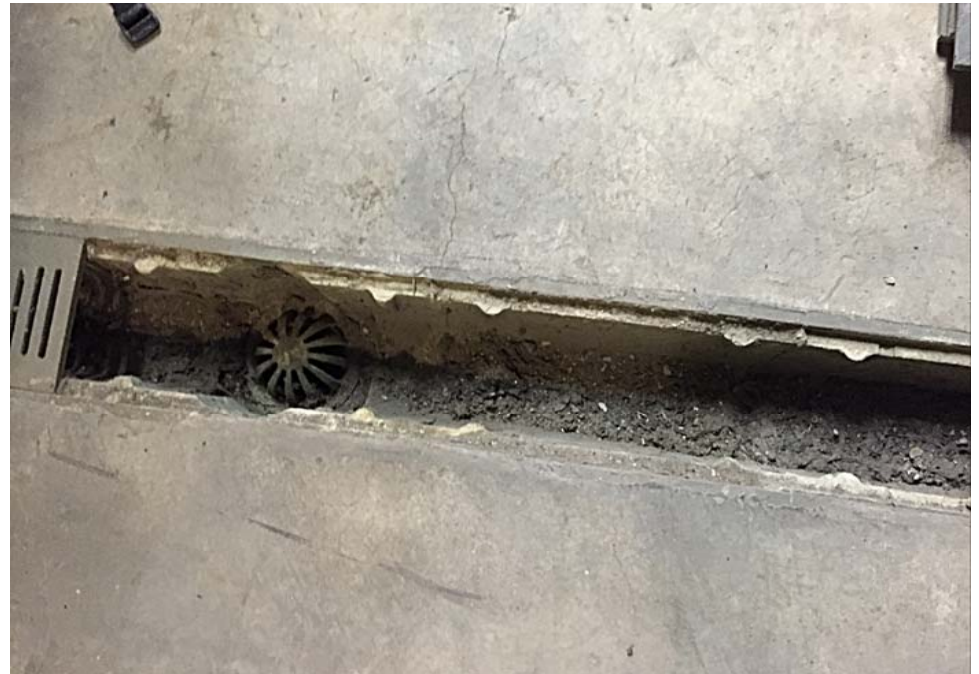
Trench Drain Before Cleaning
