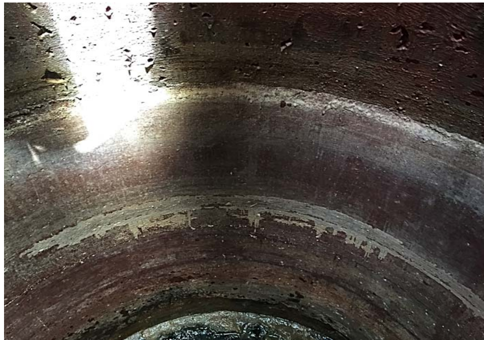
East Tank Walls Following Liquid Removal
