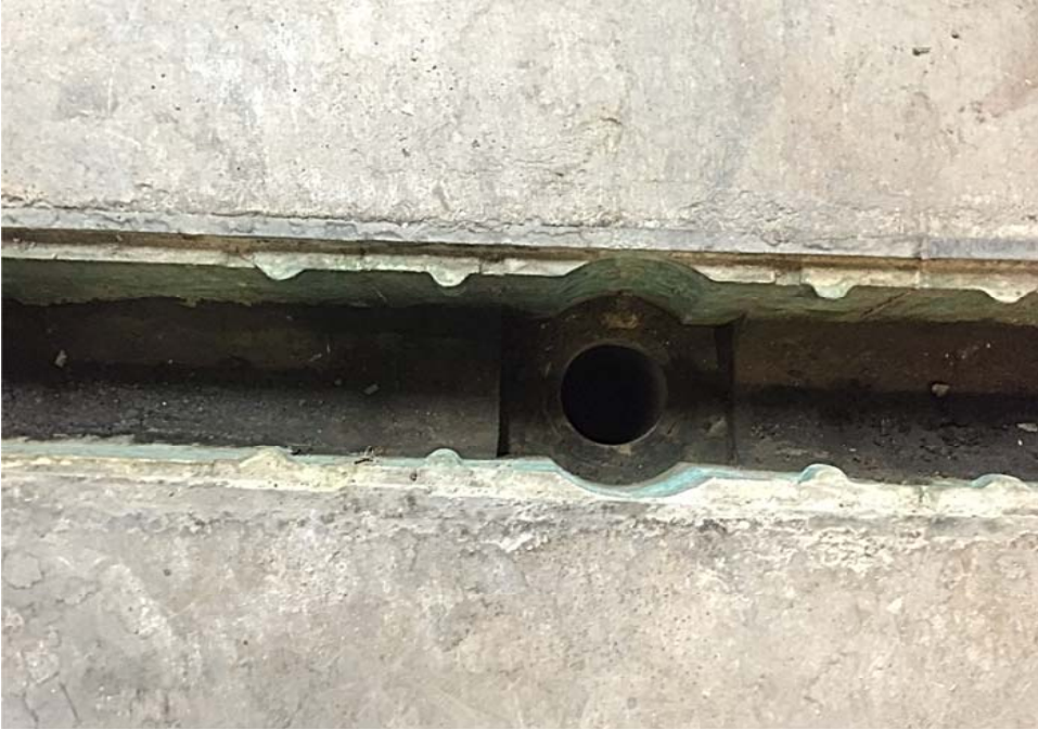
Trench Drain After Cleaning
