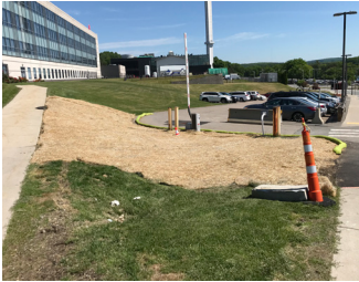
Minimize disturbance of steep slopes
