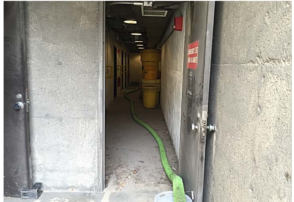
Drain Jetting and Vacuum Truck Activities
