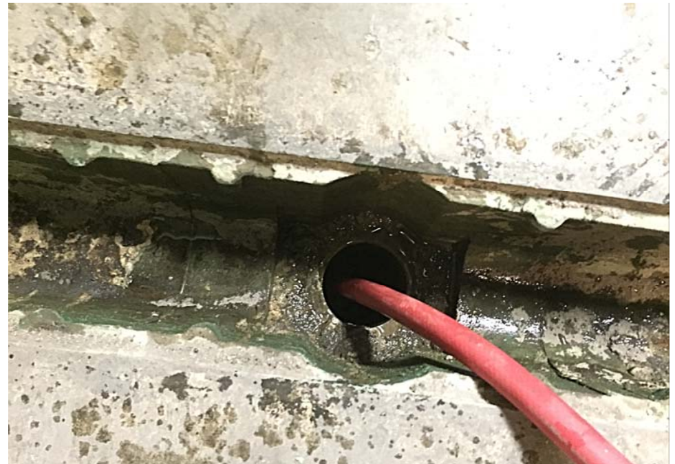
Drain Jetting Process
